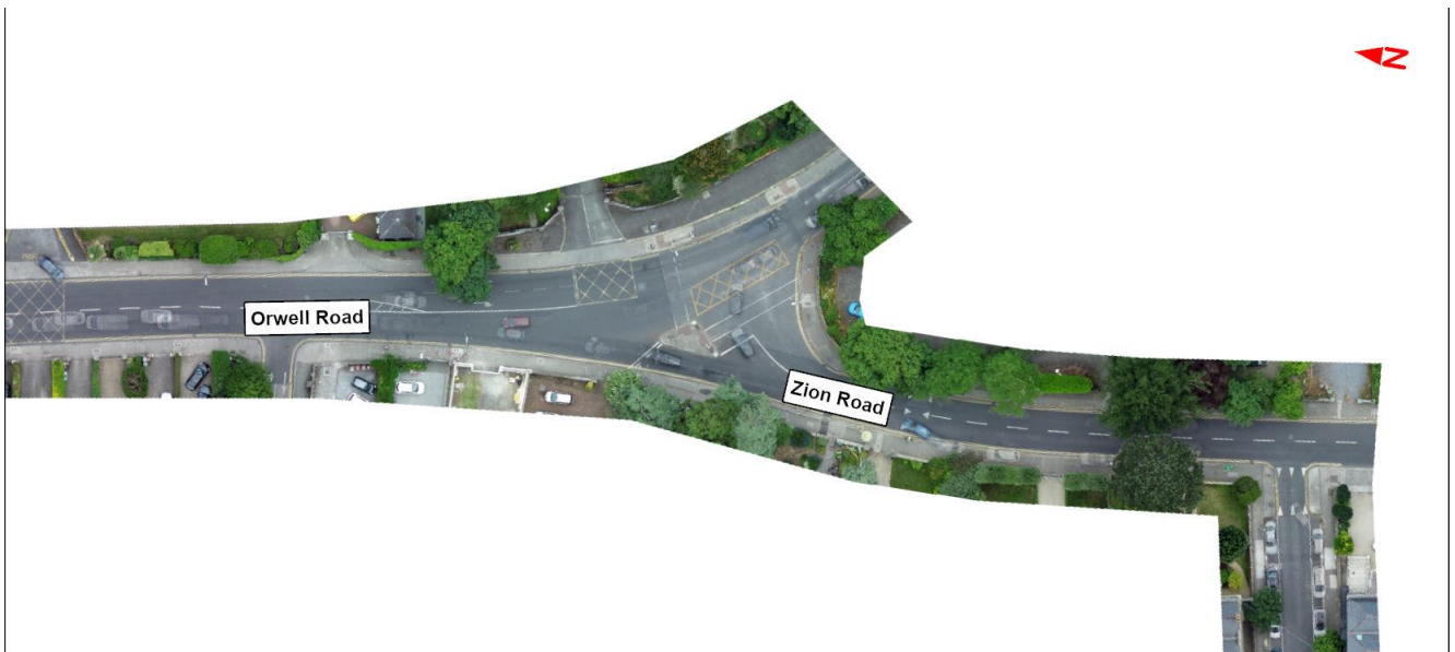
Image 5.15: Orwell Road / Zion Road Signalised Junction
