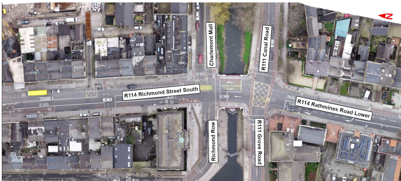
Image 5.27: R114 Rathmines Road Lower / R111 Grove Road / R111 Cheltenham Place Junction and R114 Richmond Street South / Charlemont Mall / Richmond Row Junction
