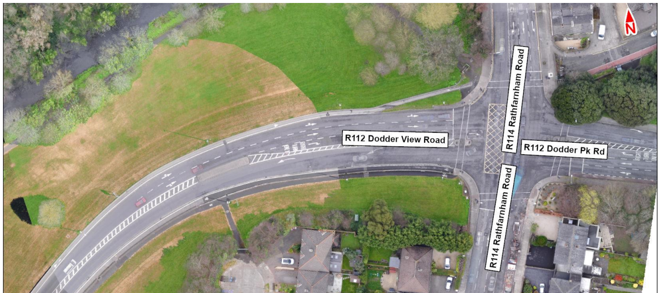
Image 5.12: R114 Rathfarnham Road / R112 Dodder Park Road / R112 Dodder View Road Junction
